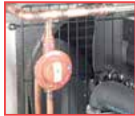
HEAD PRESSURE CONTROL (FLOODING VALVE)
