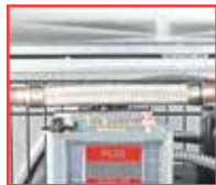
LIQUID LINE VIBRATION ABSORBER (SEMI-HERMETIC ONLY)
