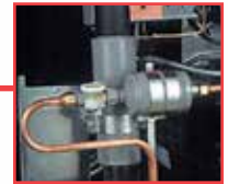
LIQUID LINE FILTER/DRIER
