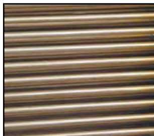
Close up of "bare tube" condenser.
