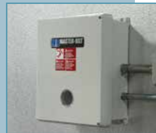
Other boards for plasma and storage freezers are mounted on the outside of the walk-in in a protective housing.
