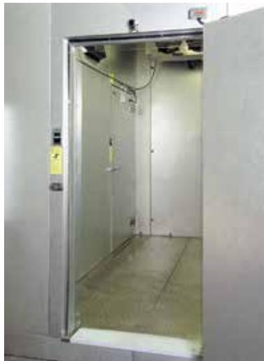
**The ante-room** reduces ice formation in plasma and storage freezers by providing a barrier between ambient air and -40°F conditions in the freezers.
