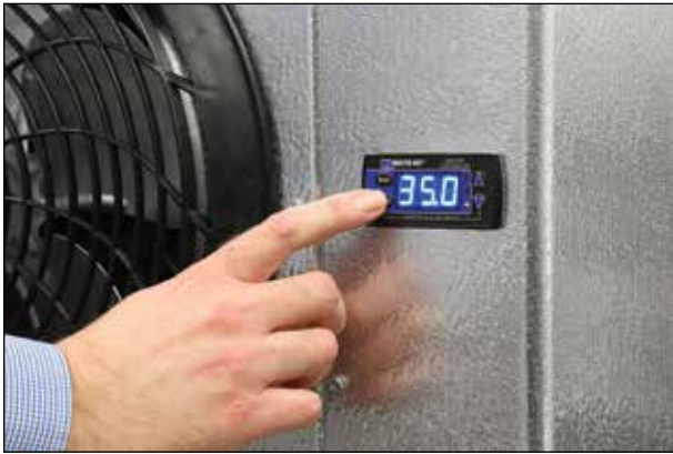
The Master Controller Reverse Cycle Defrost interface is mounted to an evaporator coil.
