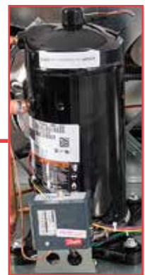
Compliant, energy efficient scroll compressors featured exclusively in low temp units for added reliability.
