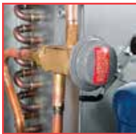
Head pressure control valve ensures proper operation in low ambient conditions.
