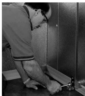
Attach slam brace with fastener provided
