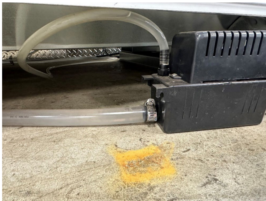
Figure 17 – Condensate pump
